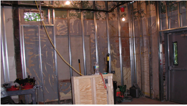
Constructing new Cook's Kitchen 2011
