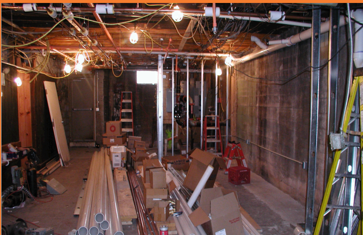
New heating system with new electric room and basement social space renovation 2011
